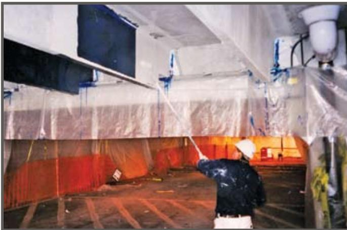
Application of a fire-rated colored coding on precast units.
