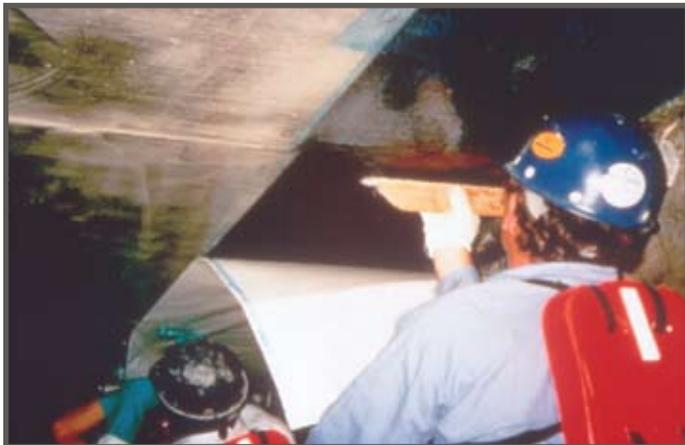
Overhead application at hospital to strengthen floor for high density filing system.
