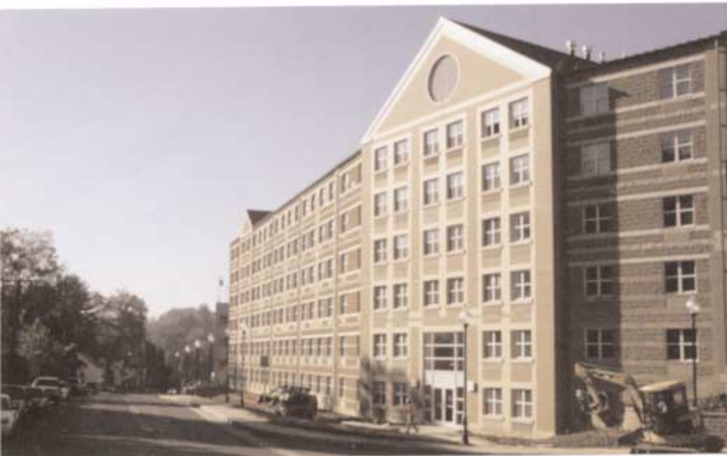
This 400-room dormitory at Fairmont State University was completed in 13 months, thanks to the design-build process. The project features precast concrete hollowcore slabs, which sped construction and saved material.
