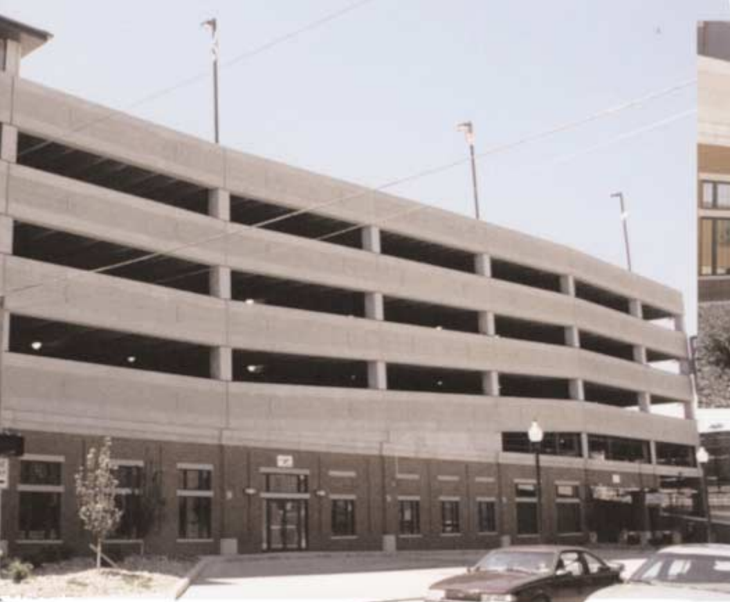
The new Parkersburg, W. Va., intermodal/mixed-use parking facility was produced on a design-build contract. It features an all-precast concrete structural system that helped meet the deadline and budget.
