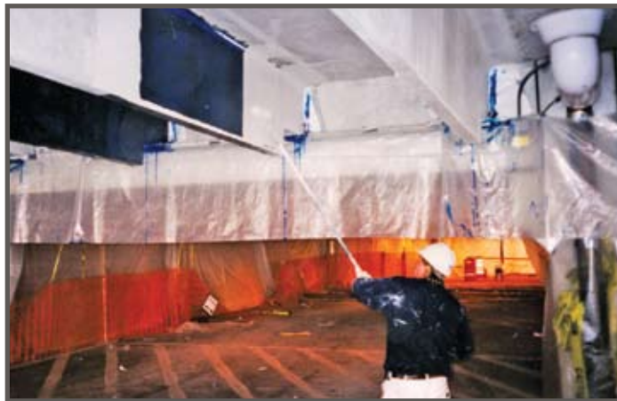
Application of a fire-rated colored coding on precast units.
