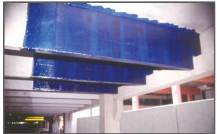
Application at precast double tee stem ends.
